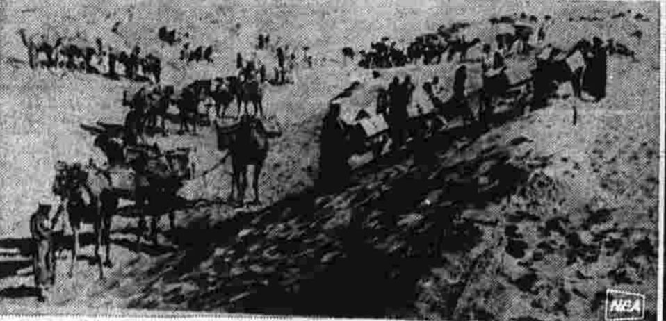
CONVOY OF CAMELS, backs laden with heavy baskets, is led to construction site.
